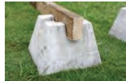
Modifying block to accept 45mm wide timber
