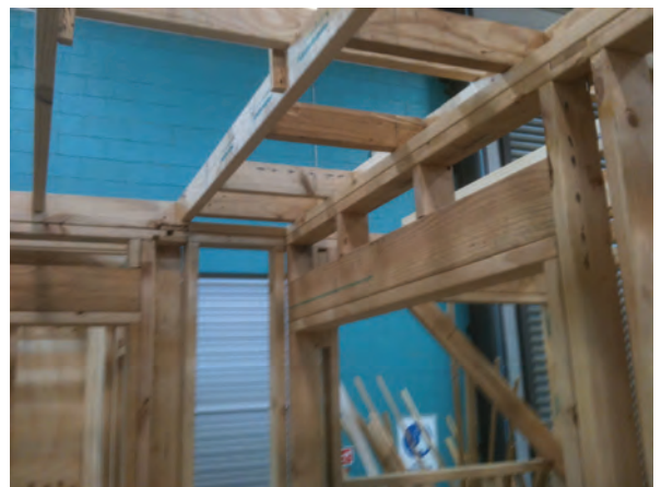
Traditional timber lintel
